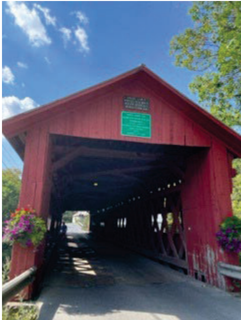
Bridge 10, taken on 9/6/2023
