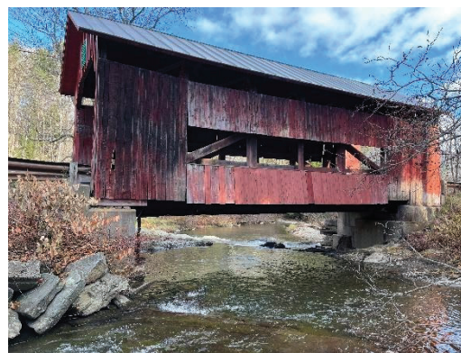
Upstream Elevation Looking East
