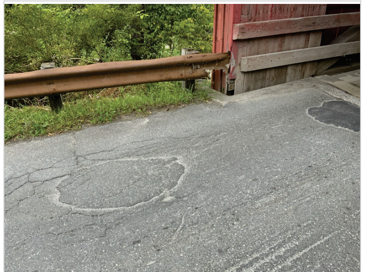
Abutment 2 transition rail
