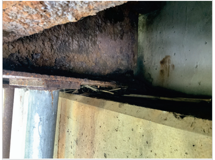
Beam 2 abutment 2 end
