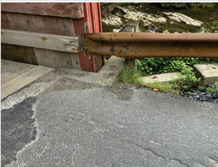
Abutment 2 transition rail
