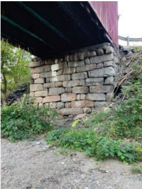
A picture of the underside of bridge 10, taken of 9/6/2023
