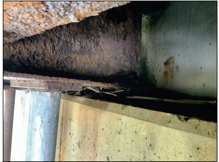
Beam 2 abutment 2 end
