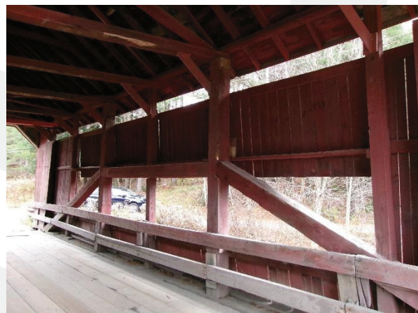
West Queenpost Truss
