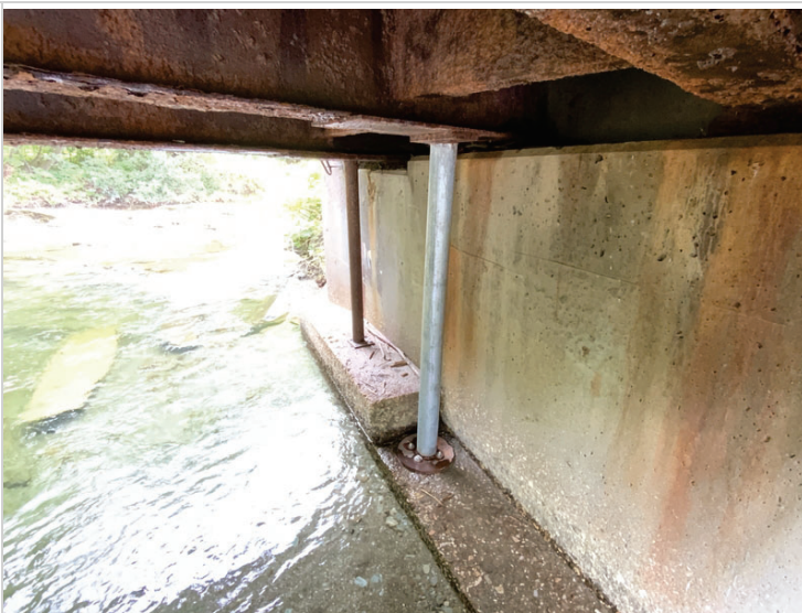
Beam 2 abutment 2 end
