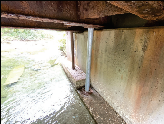
Abutment 2 beam ends
