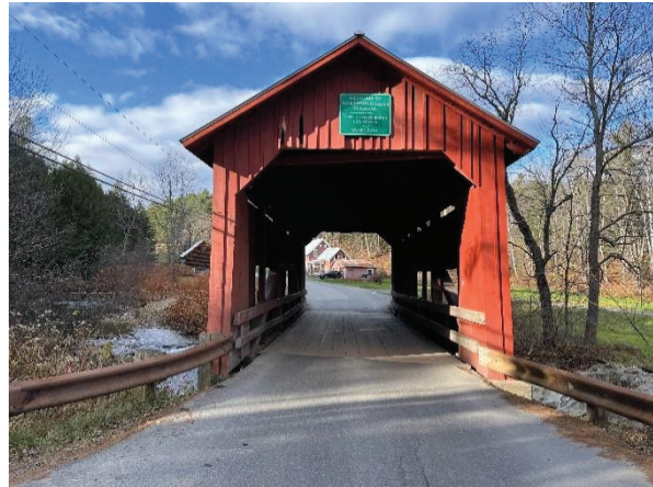
South Portal Looking North
