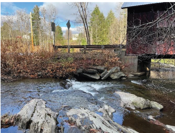
Upstream Channel with Exposed Bedrock
